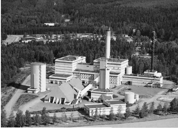
Karlskoga WTE-Plant, Sweden
